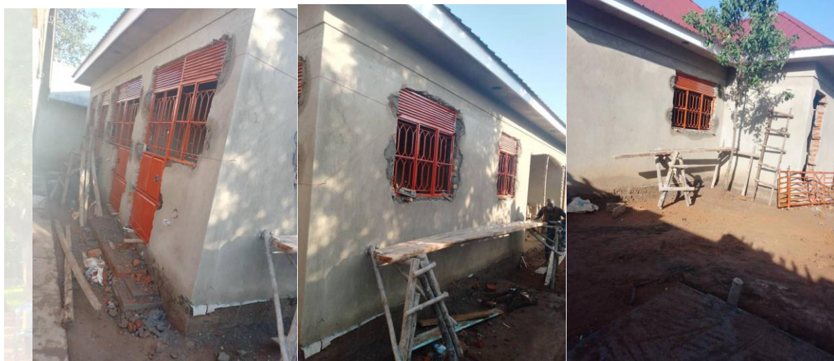
Renovation work on the building
