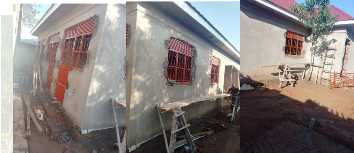
Renovation work on the building
