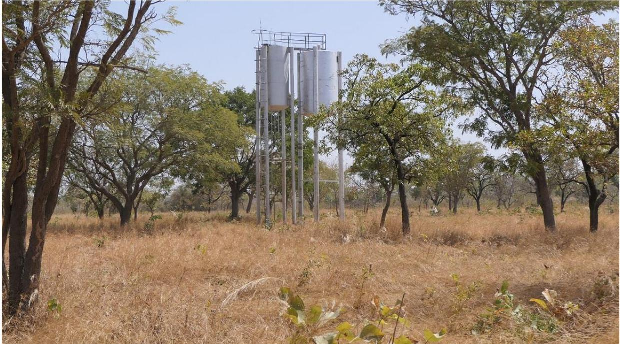
We have added a new 20m<sup>3</sup> water tower. The available water volume is now 32m<sup>3</sup>.
