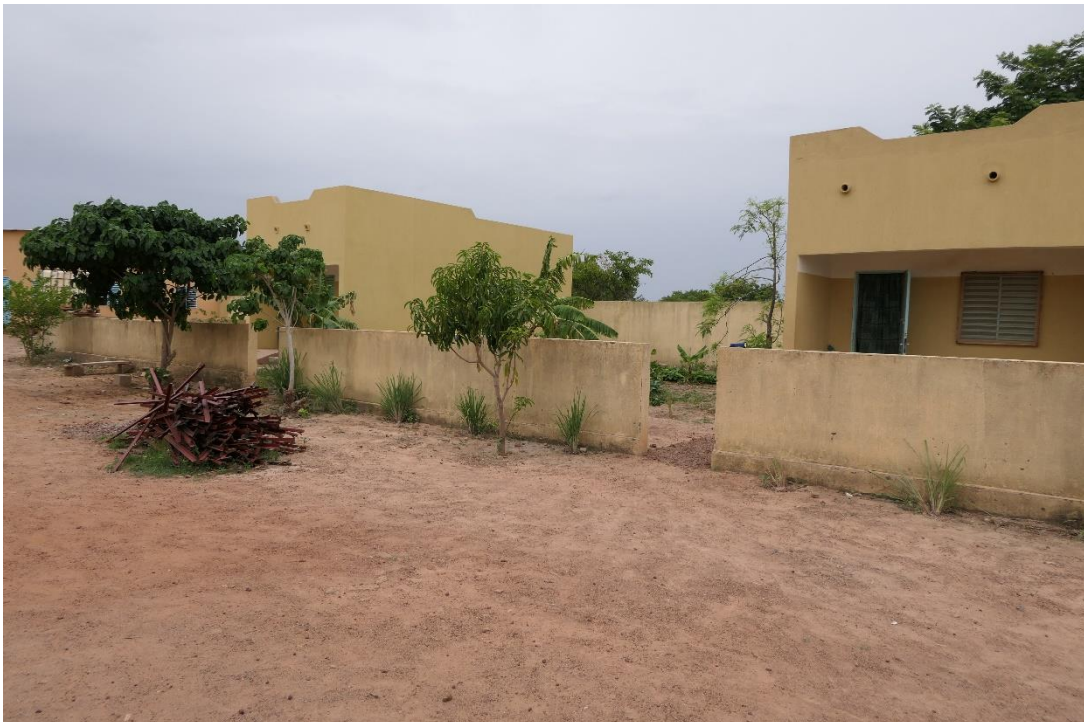
Houses for supervisors at the boys' foyer
