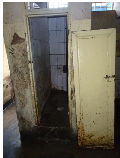
A toilet in the detention center
