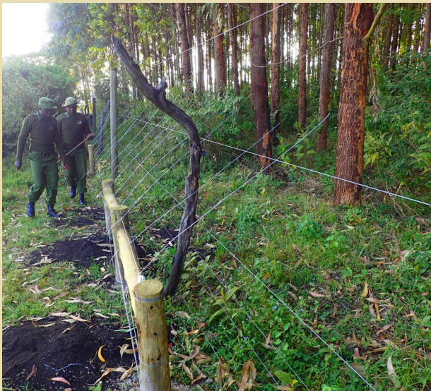
Figure 9. Elephant fence construction along conservancy's northern boundary.
