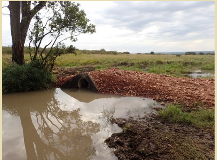
Figure 9. Newly installed culvert connecting Enonkishu to neighboring conservancy for all-weather access.
