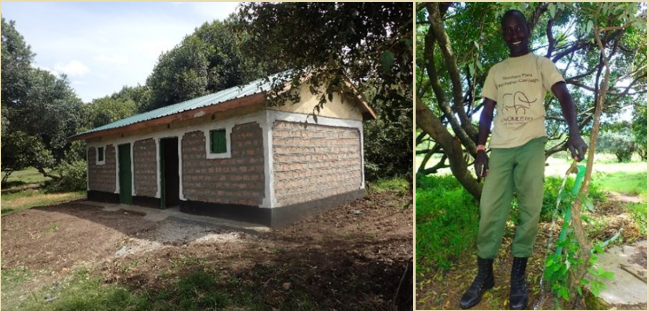
Figure 7. New construction at ranger outpost Chali Chali, including 2 bedrooms and piping water closer to the living quarters.
