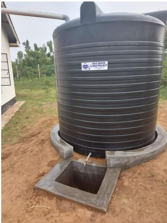
Water tank fitted on base
