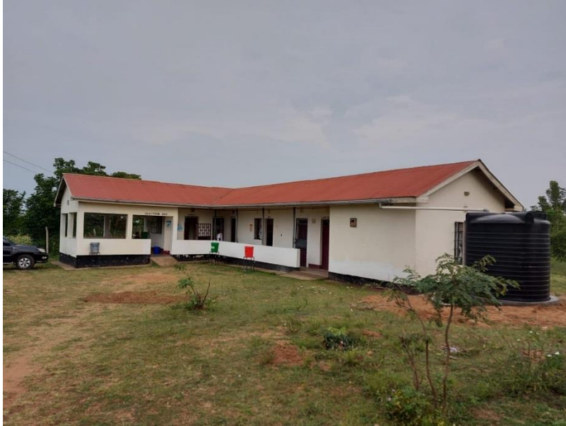
Omia Diere Health Facility with new water tank installed
