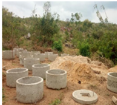
Well construction on different stages.
