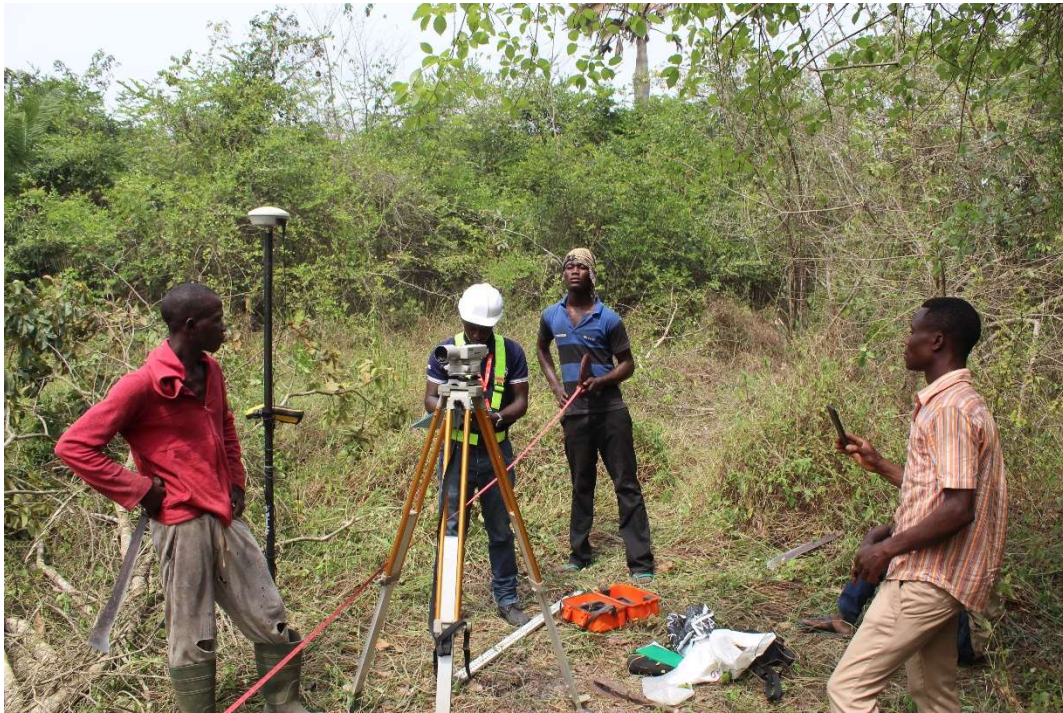
Figure 2: Leveling at dam site
