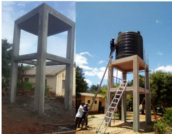
[Tower, tank, and main plumbing Installation in Mangunde]
