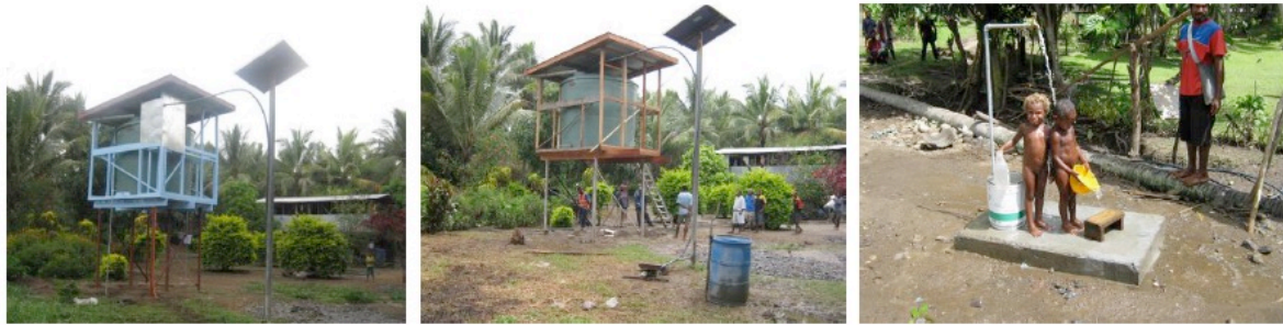
Hybrid Water Supply System – (Solar Pump & Rain Catchment)
