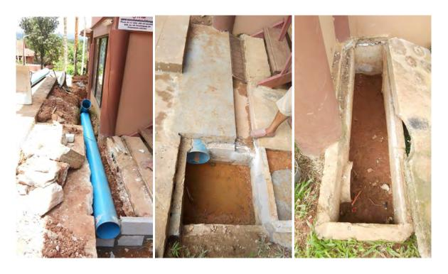
b. Installed two main lines of large PVC pipes collecting storm water and divert it away from slopes
