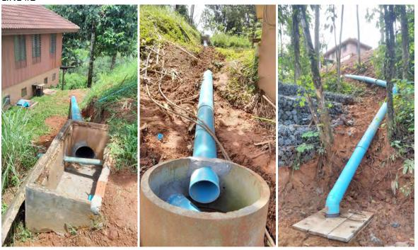
c. Install large manholes and concrete tubes under the retaining wall and service road below, to drain storm water into the stream.
