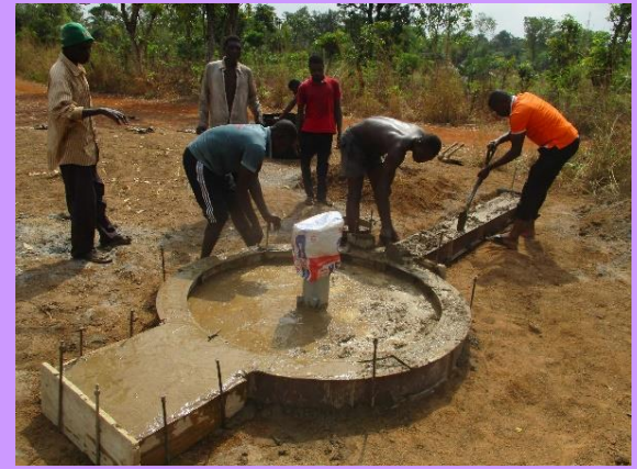
Casting platform for borehole Ngujiola, Izzi
