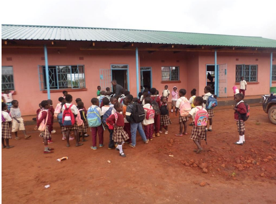
1x2 classroom block funded by EGP from UK in 2017
