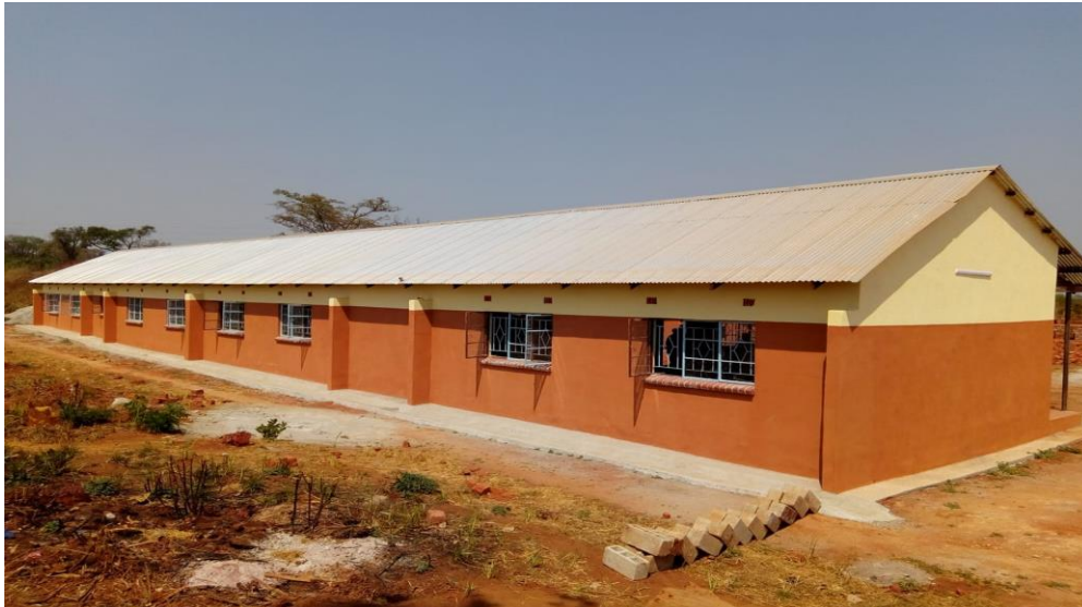
Completed 1X4 Classroom block Rear elevation funded by the Australian Embassy in 2018
