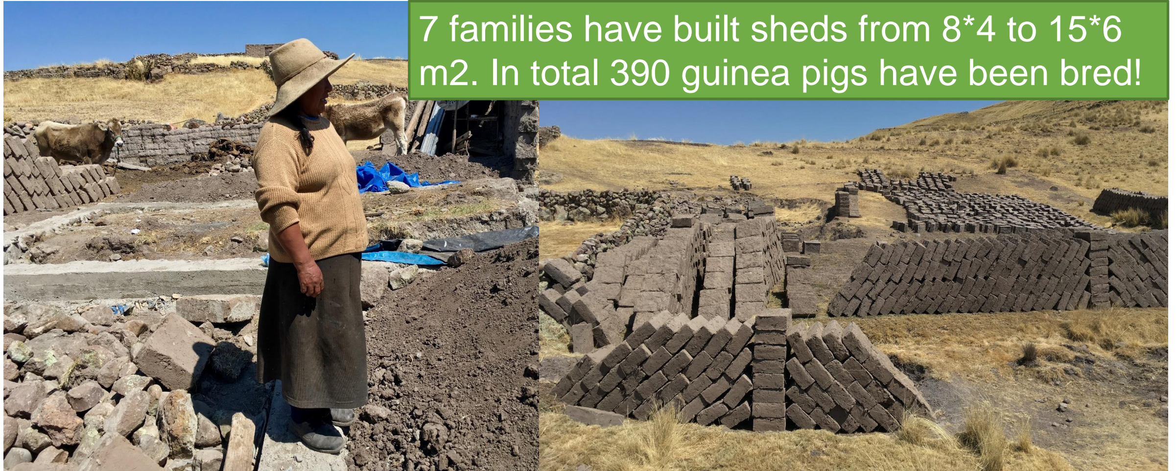
Construction of a shed using mud blocks. A sustainable and economical way to improve the quality of life.
