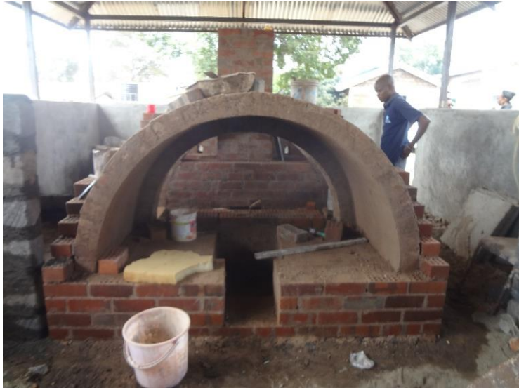
Community Cooker under construction
