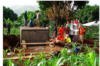
Completed storage tank
