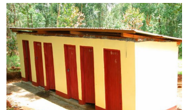
LWDGC construct new latrines
