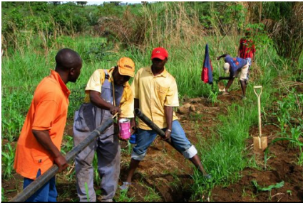
Laying the pipe into the pipeline
