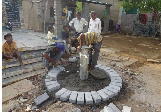
Masons are constructing the platform at village 1
