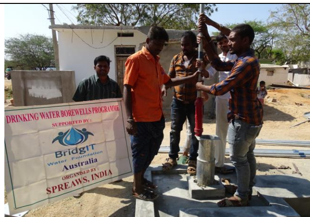
Technicians and village volunteers are inserting the G.I pipes in Peddapalle Harijanawada village
