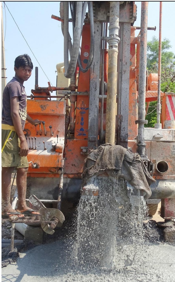
Drilling the bore in Sugalthanda Scheduled Tribal Colony
