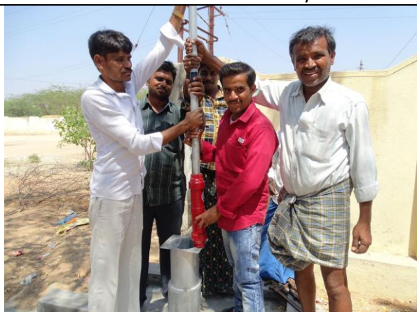
Technicians inserting the G.I pipes at Parvathareddygaripalle village
