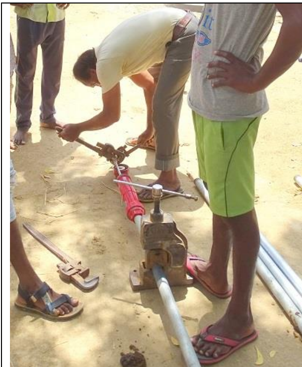
Technicians inserting the G.I pipes at Sugalthanda Scheduled Tribal Colony
