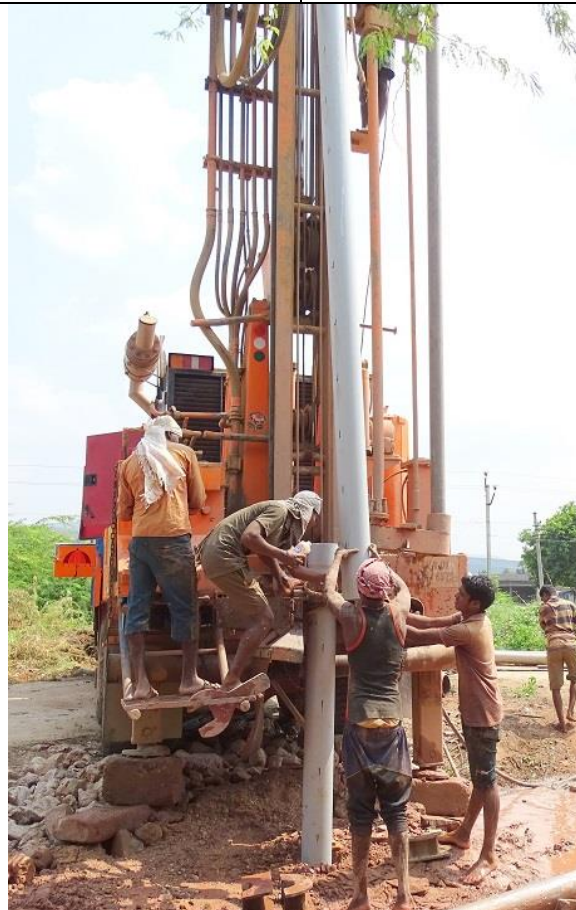
Inserting casing pipes into the bore hole at Chinna Nagireddypalle
