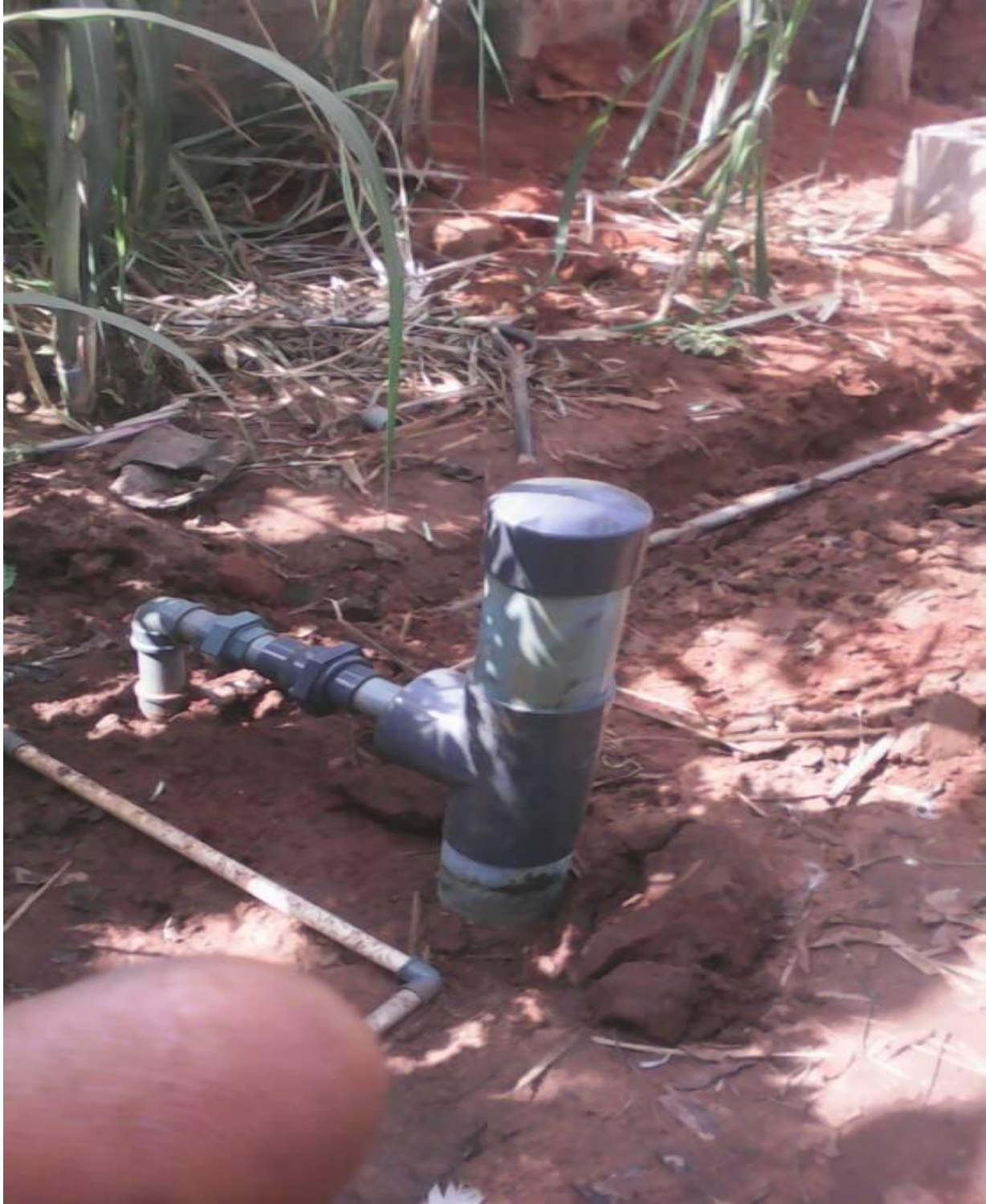
Figure 11: The artesian water source with completed plumbing installations to convey water to 40feet high water reservoir of 10,000L. This picture of the Artesian water source shows the stage where the water which flows out naturally from the aquifer layer beneath the ground had been capped. The capping further helps to increase the water pressure to flow upward and prevent water wastage. See attached video of the uncapped stage for details.
