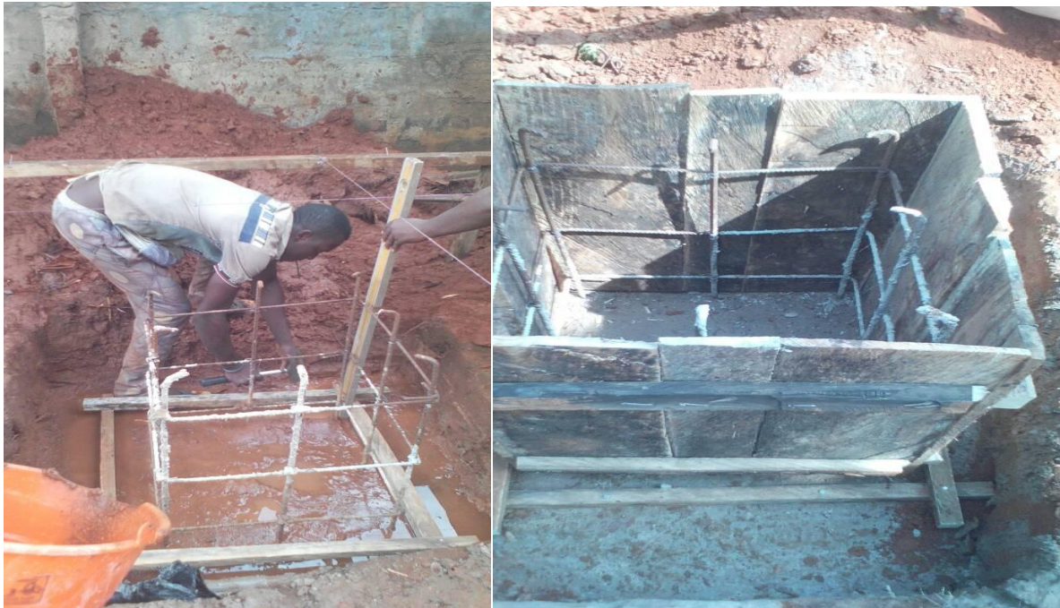
Picture 6 and 7: Construction of Basement for Water Scaffolding (continuation).
