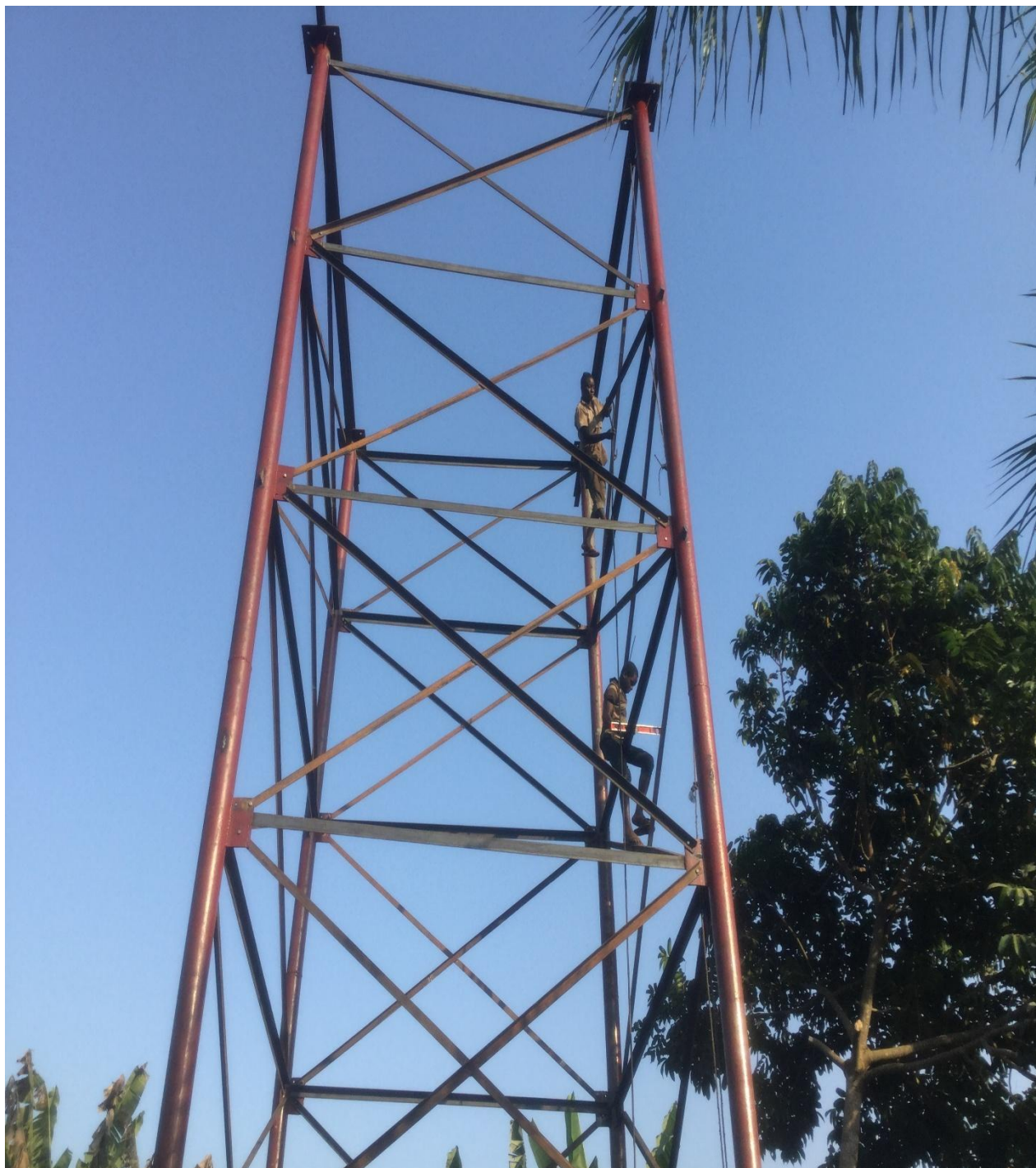
Figure 12: Ongoing construction of a 40feet high steel scaffolding to hold 10,000L water reservoir, Iyerekhu, Edo State.
