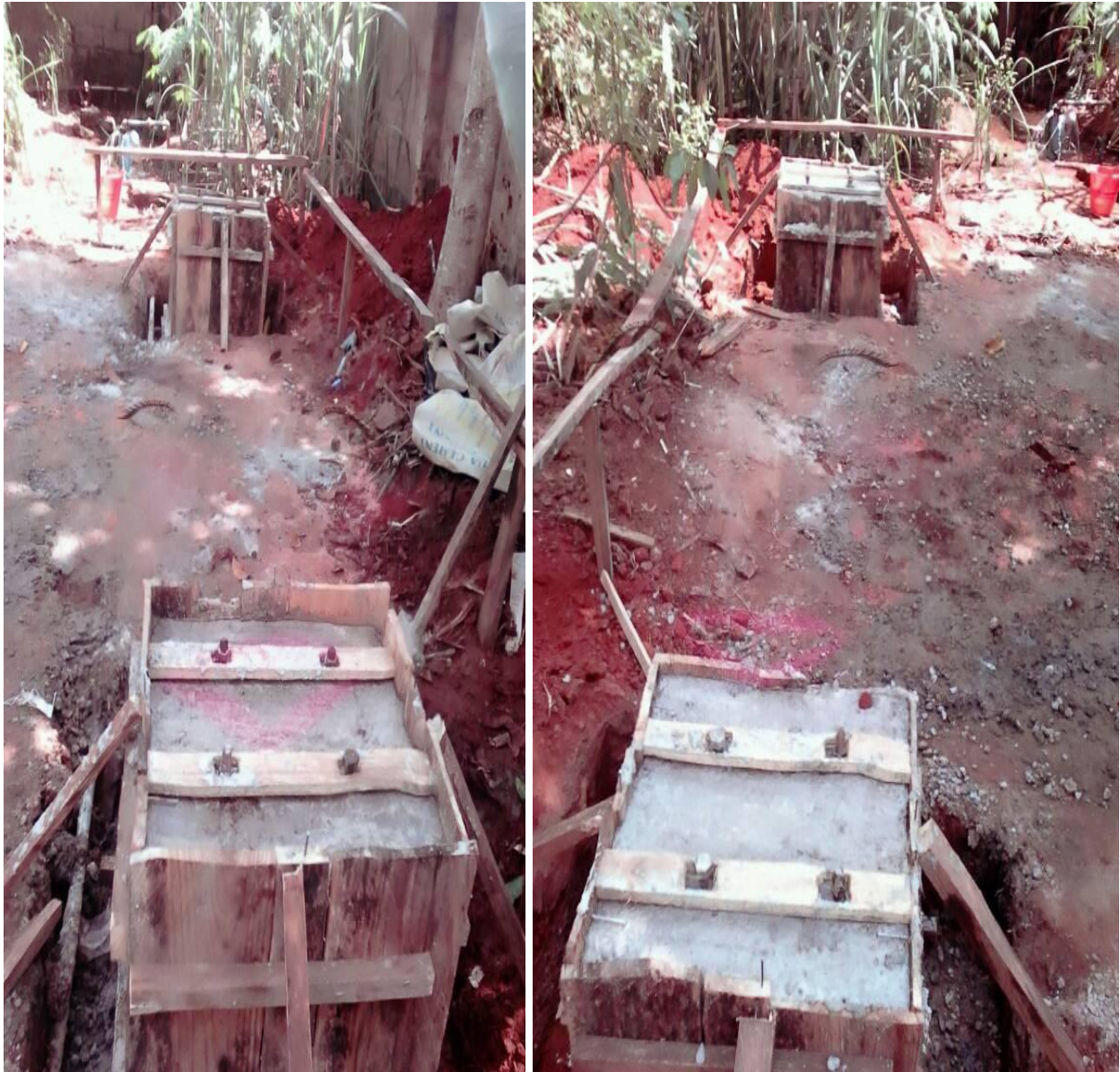
Figure 8 and 9: Construction of a concrete basement to hold 10,000L of water Storage.
