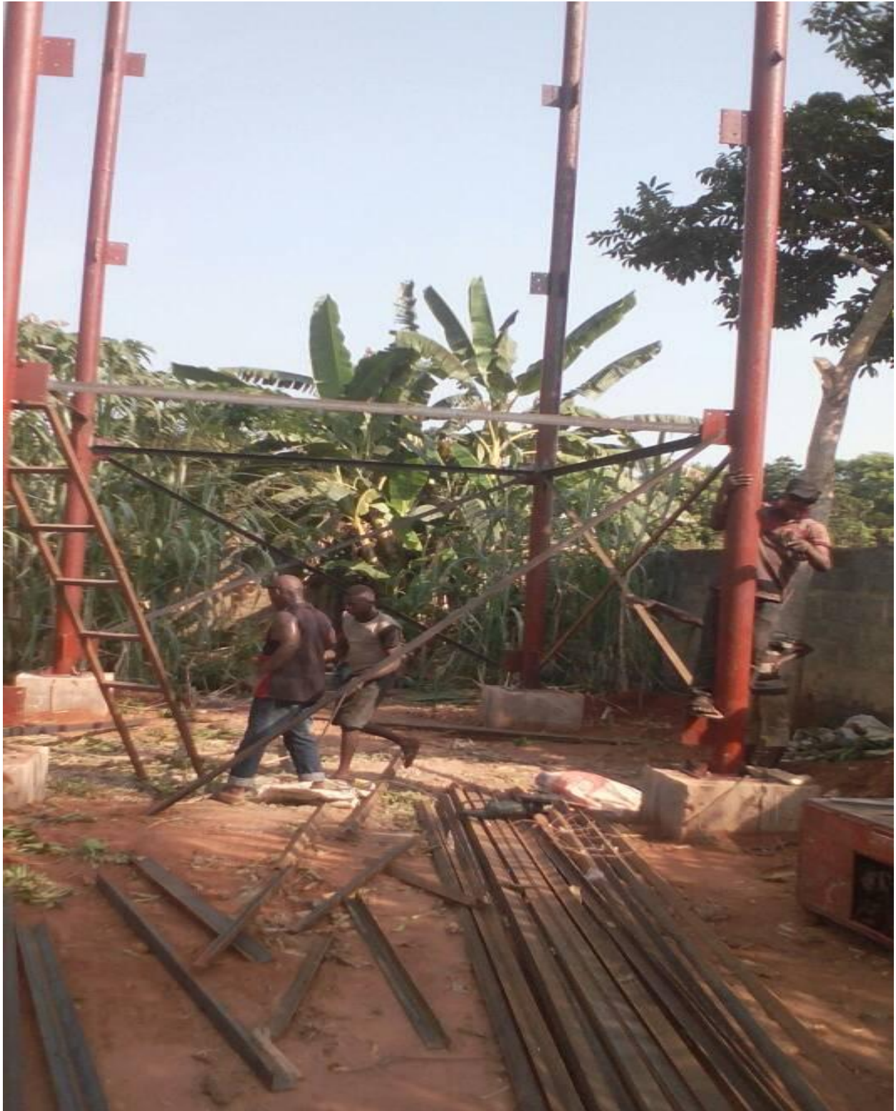
Figure 10: Ongoing construction of the 40ft high water scaffolding.
