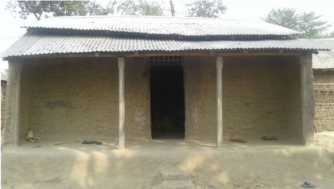
-The look of stage-one of plastering of the houses
