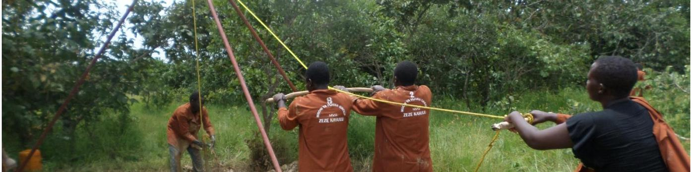
Smashing drilling taking place at Zeze in 2016 whereby the borehole of 24 metres was dug by MVG for the first time - field picture
