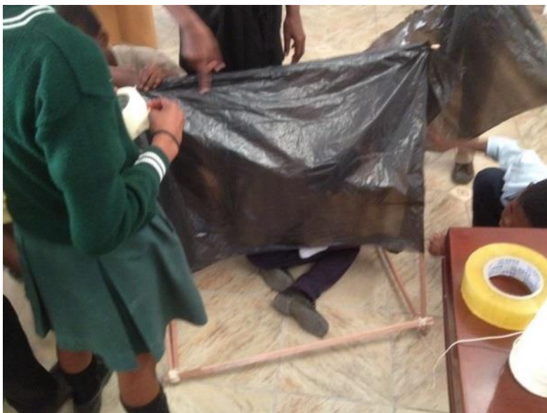
Use garbage bags to form the walls of the life-size emergency shelter
