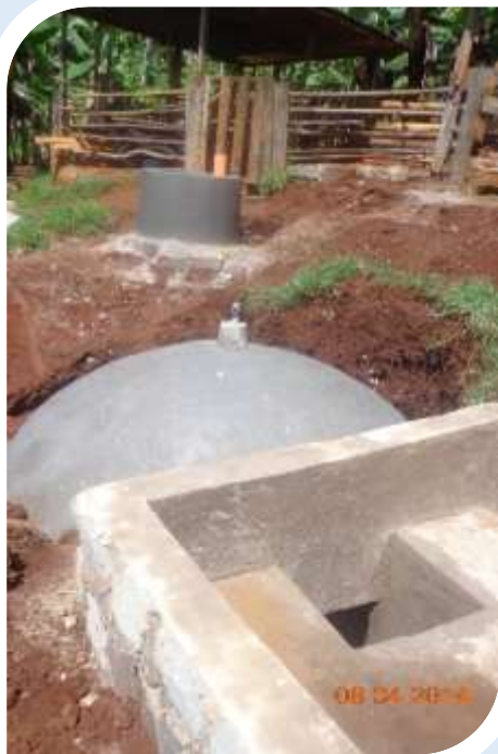
Fixed dome biogas units and Tube biogas installed by KSEI in households.
