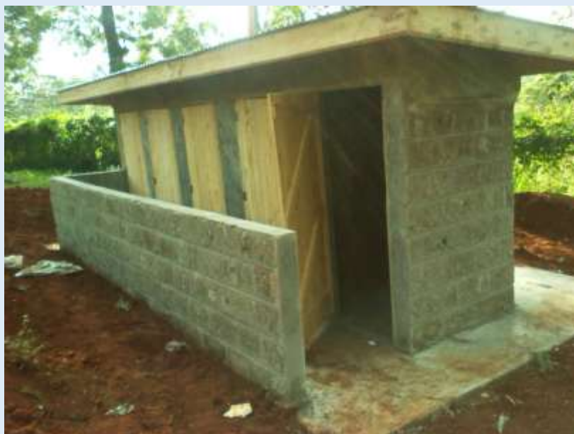
Ventilated Improved Pit Latrine constructed in a local school
