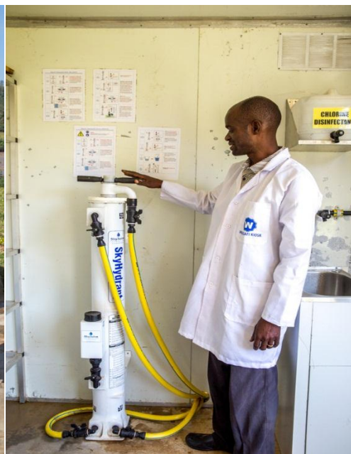
Water filter chamber at the kiosk
