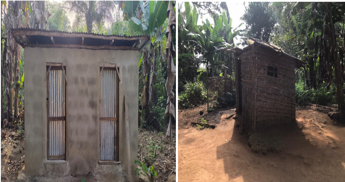
Fig 6: Latrine constructed in Tengbelor and Mogbencha respectively
