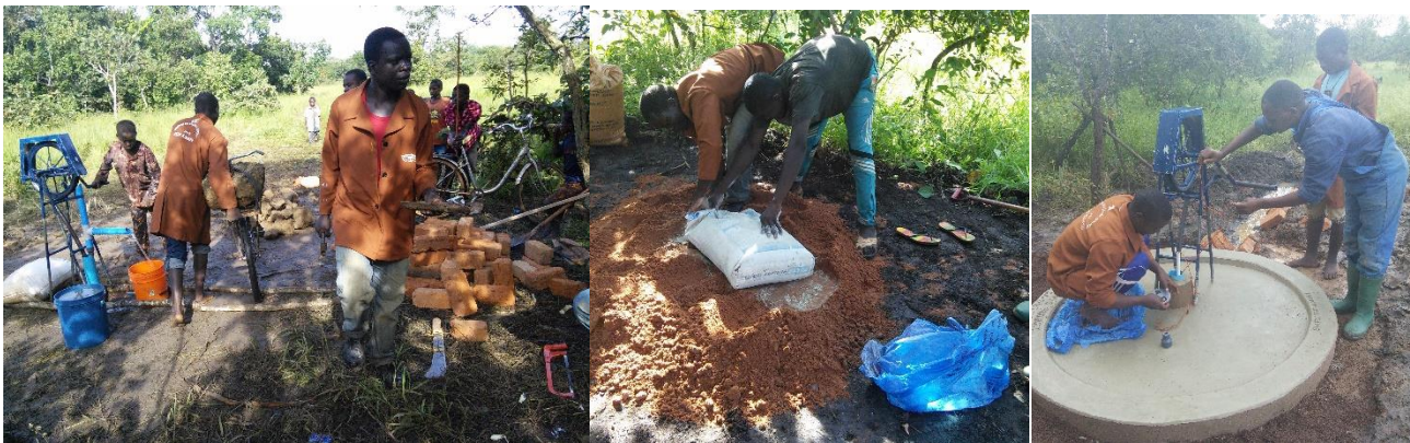
Plate 5: MVG in Processes and steps of well structures and gutter construction after reaching the water
