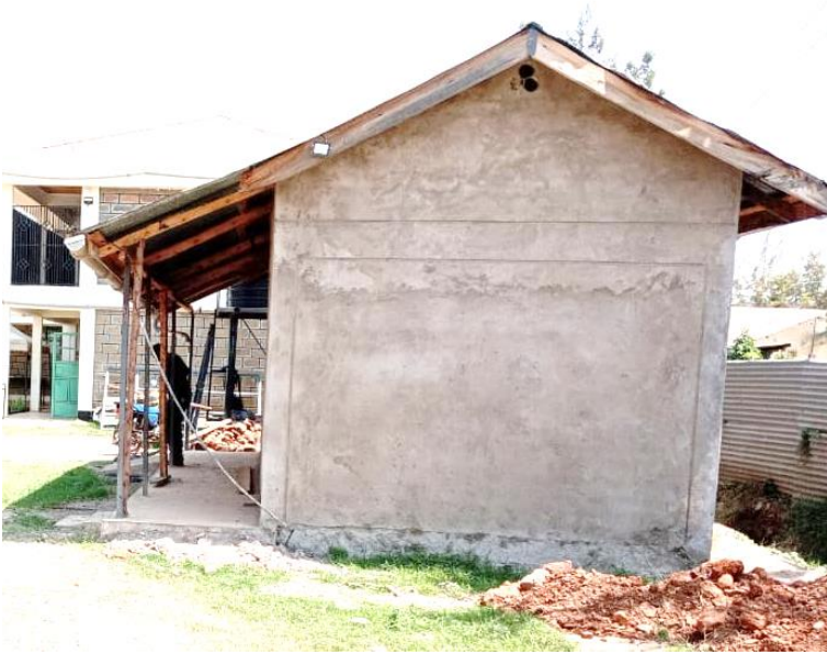
Work in progress – changing the wall from iron sheets to brick walls.
