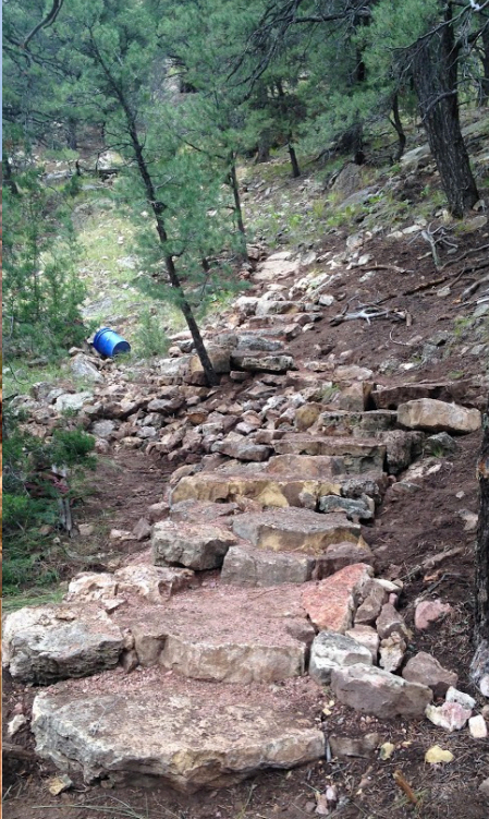
Making sustainable climbing access with rock steps.
