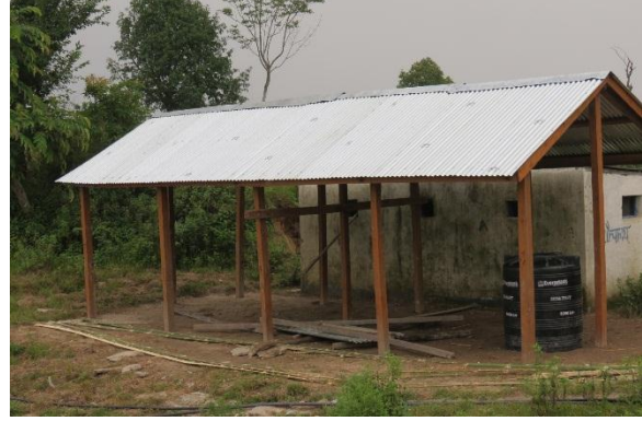
Figure 11 TLC: Bhuwaneshwori Primary School, Dadakharka, Under Construction
