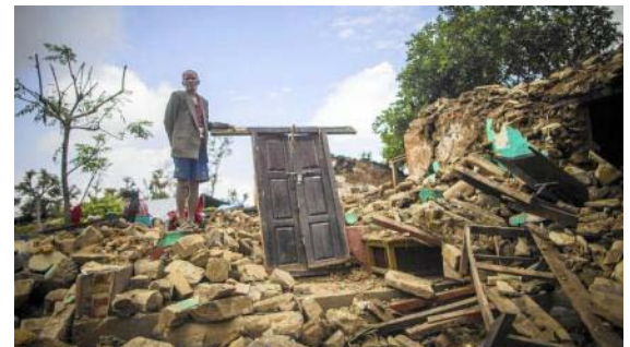
Destroyed house in Gorkha District. (web)
