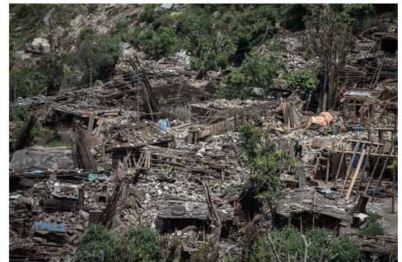
Destroyed rubble stone houses. (web)
