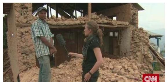
Collapsed house showing horizontally bedded rubble stone construction in Gorkha District. (web)
