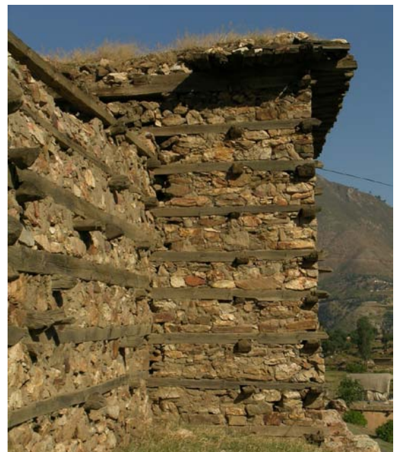
A 19 th century timber-laced rubble stone fort in Northern Pakistan near epicenter of 2005 earthquake that killed 89,000 people. It survived with very little damage despite having been abandoned and unmaintained for half a century! (Photo by author)
