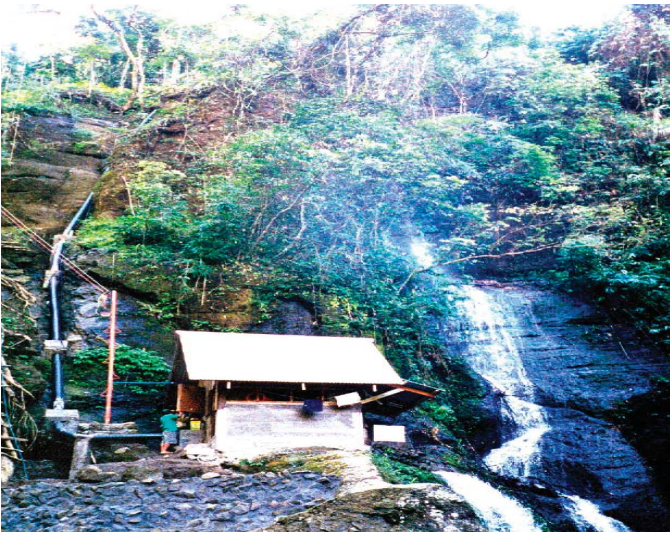
Operational SIBAT Micro Hydro project in the Philippines
