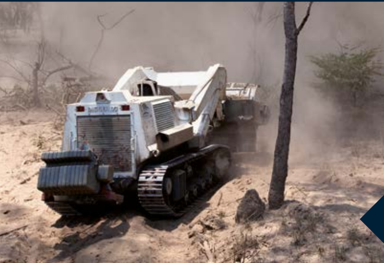
Digger Mechanical clearance, Mozambique
