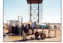
The community has four public water stations, consisting of deep wells and pumps that bring water to elevated storage tanks from
