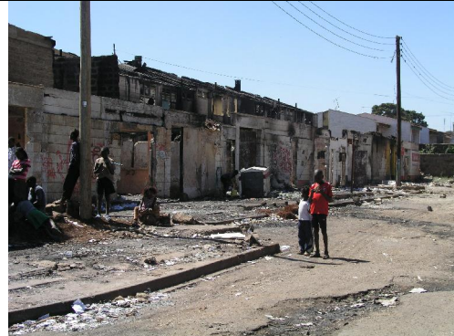
Empty shell: shops & homes burnt down
