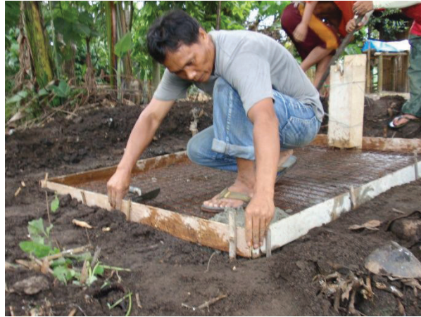
Figure 16: Tap Stand Construction with Dadz
