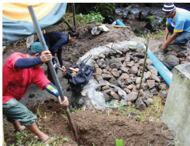
Figure 6: Catchment Tank Foundation
