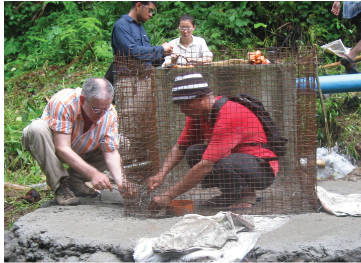
Figure 7: Catchment Tank Framing
