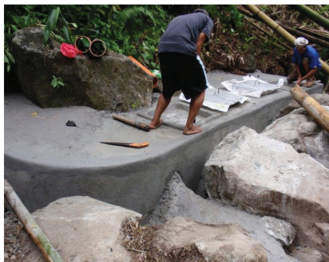
Figure 12: Completed Impounding Tank
