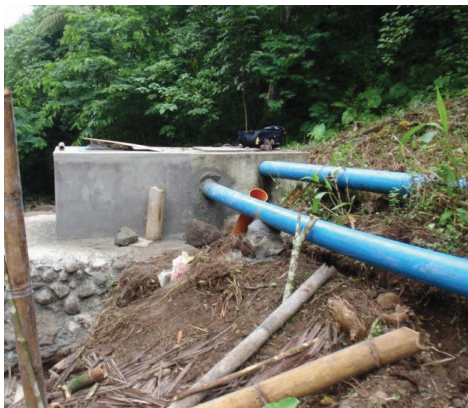
Figure 8: Finished Catchment Tank
