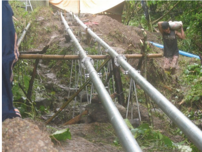
Figure 10: Drive Pipes
