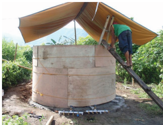
Figure 15: Reservoir Construction
