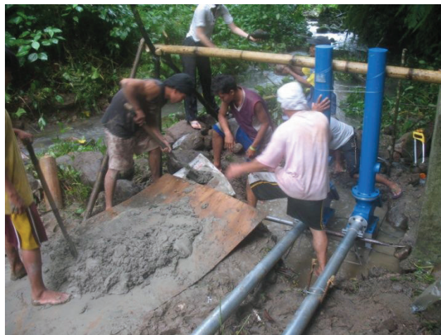
Figure 9: Ram Pump Placement
