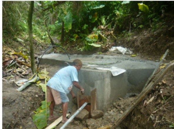
Impounding nearly finished
