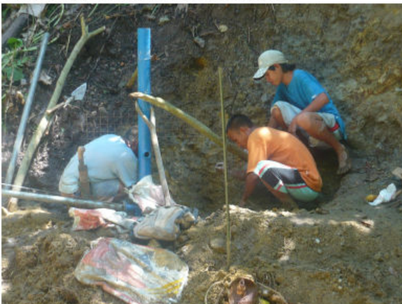
Installation of ram pump
