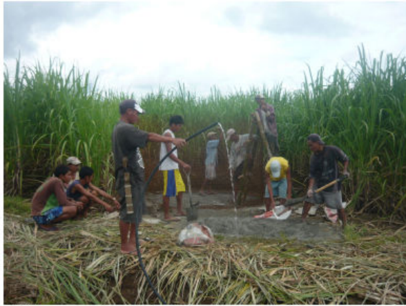
Water pumped up by the first ram pump used for construction of 10.000 liter reservoir.
