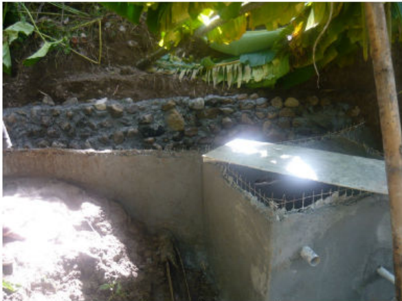
Impounding and catchment under construction
