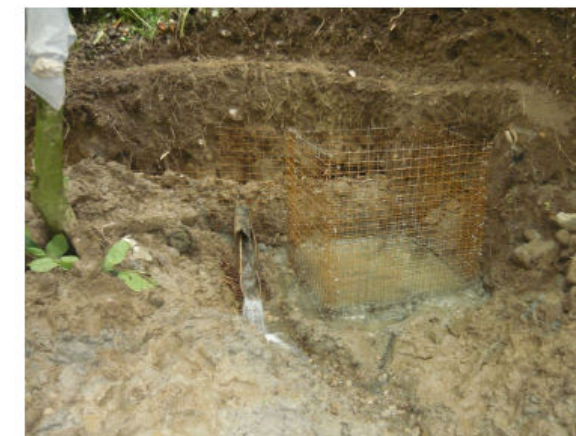
Start of construction on impounding and catchment
