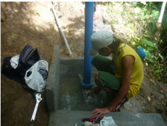
Local Technician with ram pump
