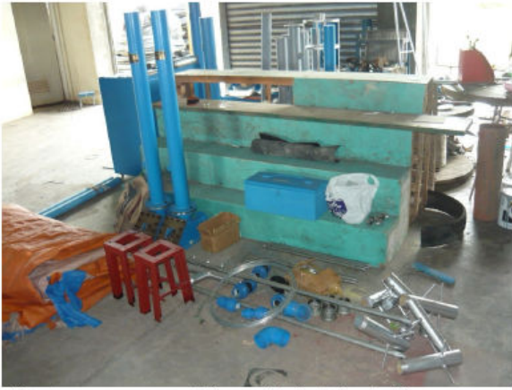
The two ram pumps and the pre fabricated materials
