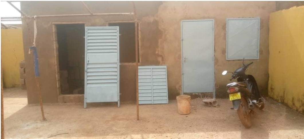
Construction of the 2nd workshop and their openings (doors and windows)
