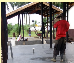
New Construction Ebola Surveillance Station
