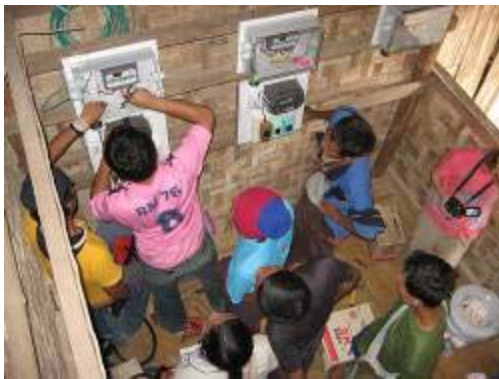
Medics work on the charge controllers and inverters in the equipment room
