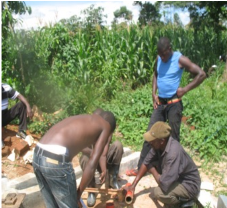
The borehole mechanic assembling a new borehole in Lukalu.
