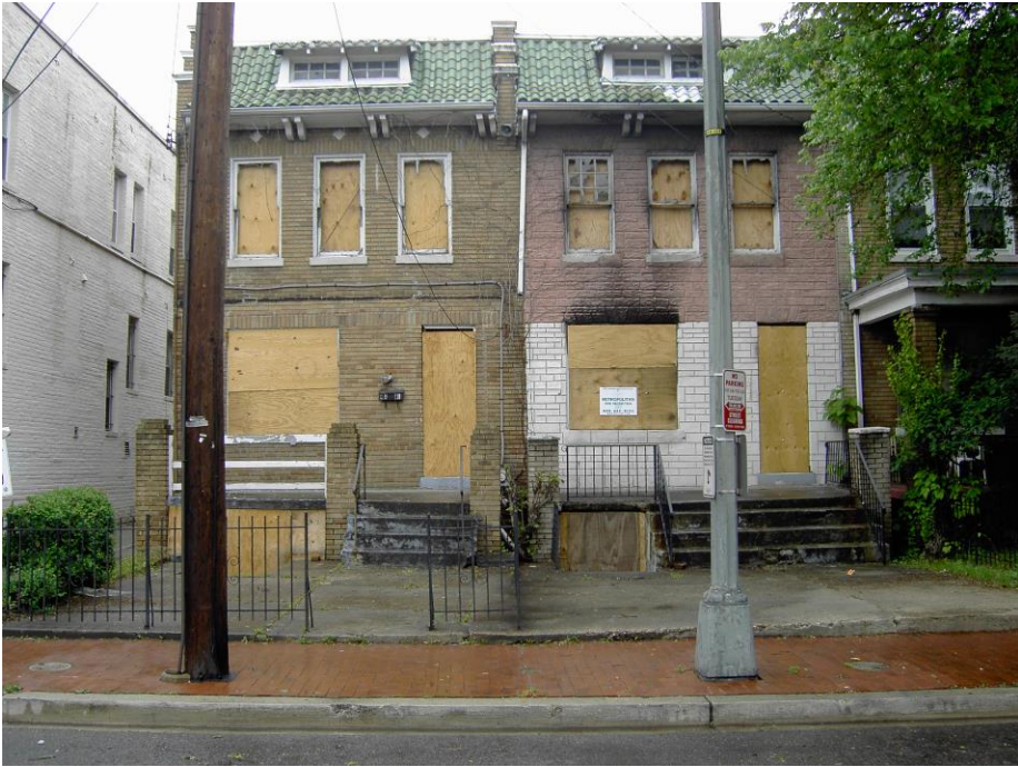
Photo: As-is property, as seen from Kennedy Street, NW.
