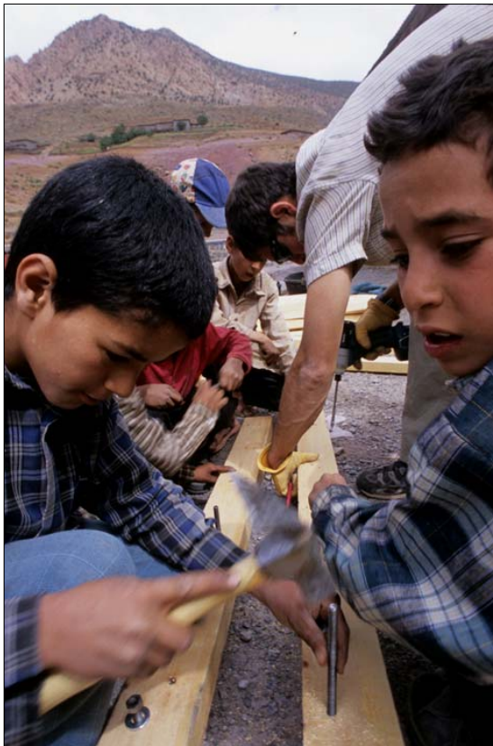
Students help build rafters for their new school roof.
