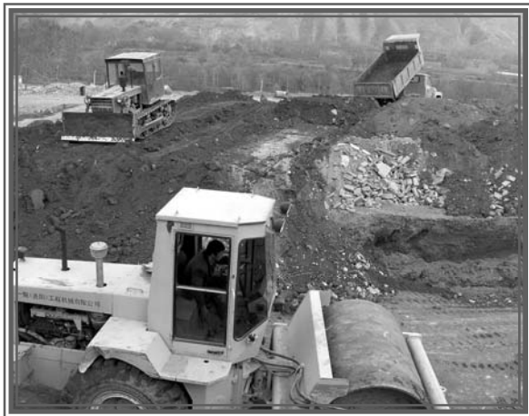
In 2006, land was broken in the construction and restarted in April 2007 after the winter season.
