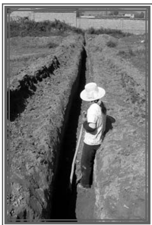
Digging a hole for the ground work of the outer wall.
