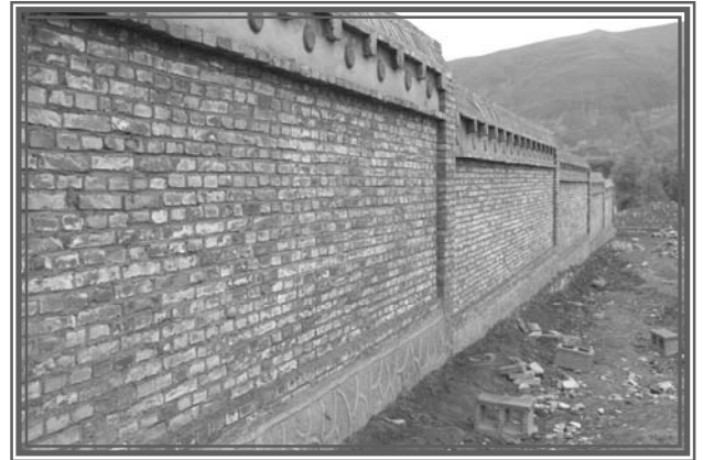
October 2006, Birth Center construction of the outer wall.
