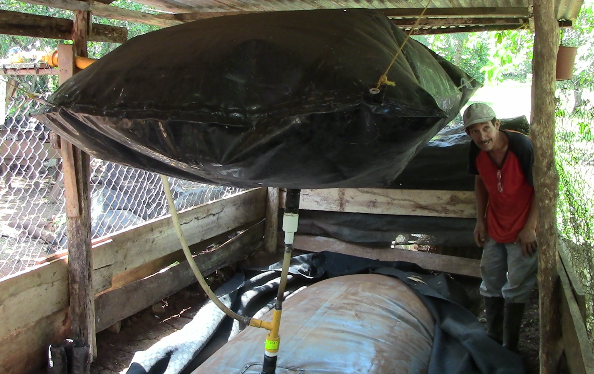
Juan Nicaragua is about to start walking on his biobolsa to agitate the bladder containing the manure and water mixture so it continues to effectively produce biogas and biol fertilizer. Periodically moving the bladder around ensures effective methane gas production to feed the line to the kitchen, seen in the upper left of the photo. “Less costs, less work,” he says about Tecnosol’s biobolsa – a realization made possible with your help!
