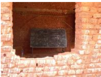
New classroom at El Tagwa School under construction.
