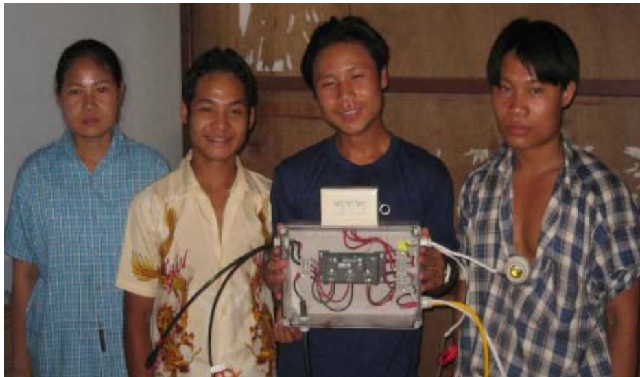
Medics have completed the wiring for a new system.
