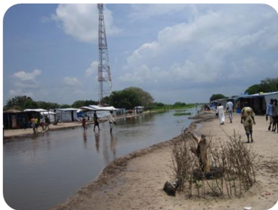
Picture 2: Ayod Market, road completely flooded.
