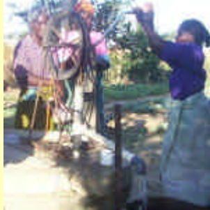
Well construction and Rope Pump
