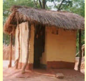
Construction of latrines.
