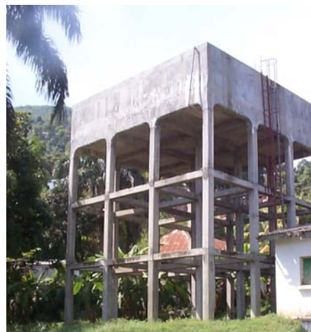
42,500-Gallon Elevated Storage Tank
