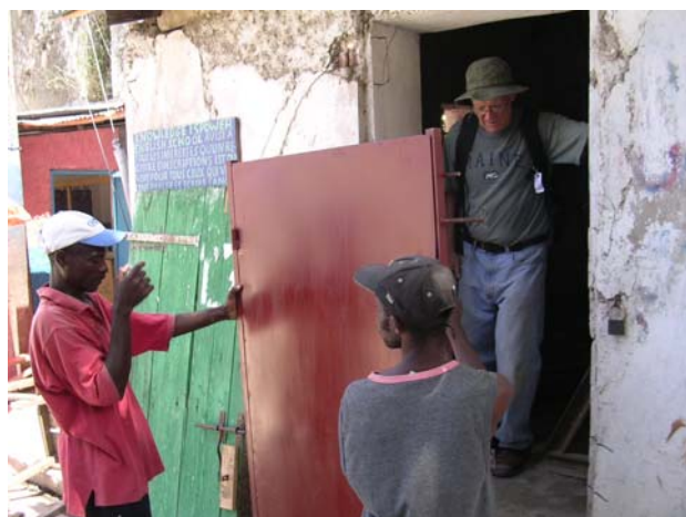
Installing New Door on Pump House to Protect Control System
