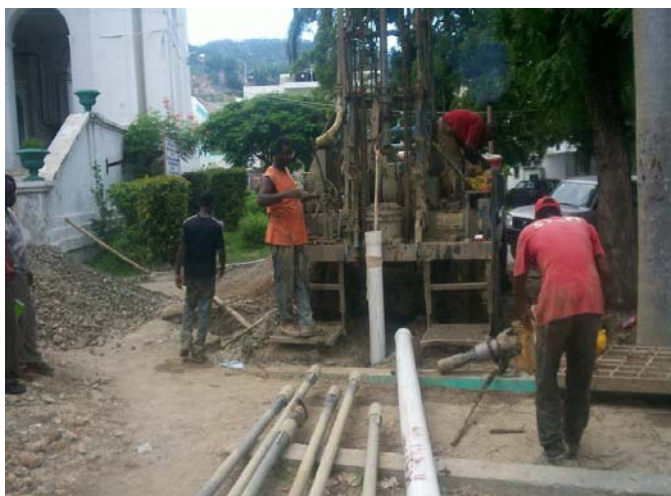
Drilling the New Well at Hospital
